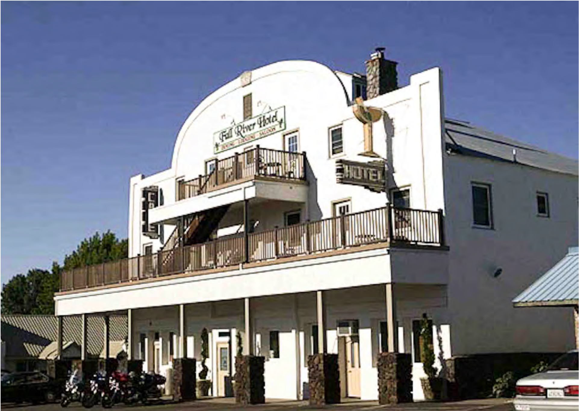
The historic Fall River Hotel. (2003)
