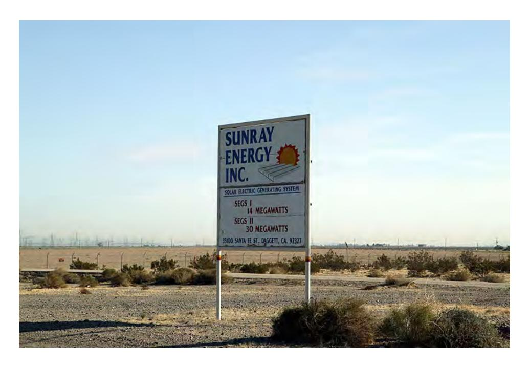
These plants reflected the sun's rays off mirrors to a boiler. That heated water in the boiler and generated electricity. (February 2006)
